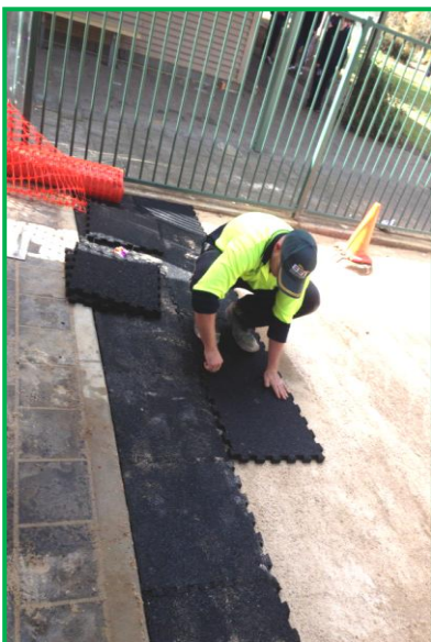
25mm Underlay installation
