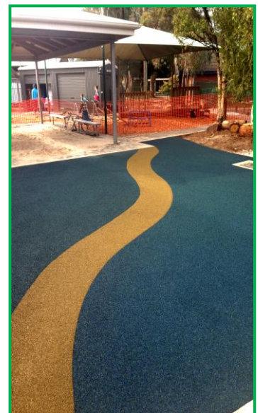
Finished Surface with a CFH 1.45M
